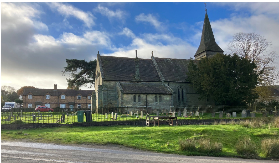
Image: St Mary's Church with the Almshouses behind
